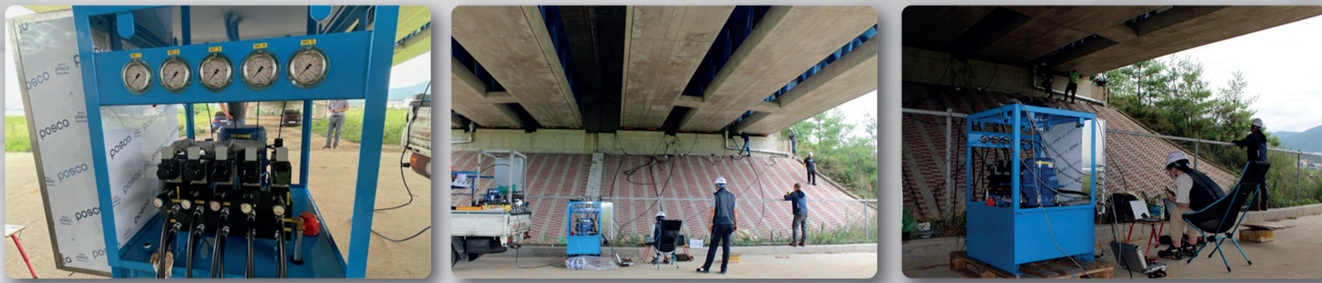
Synchronous Lift System Using Quantity Risk Analysis
